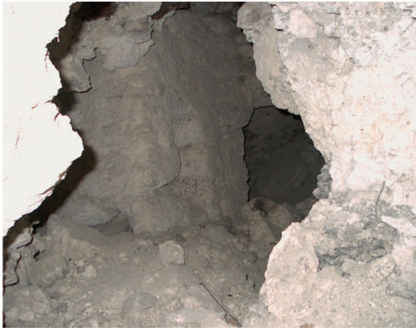
Figure 17. Buried structure in Group A
