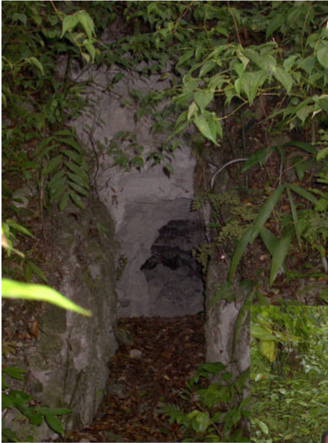
Figure 12. Looters' trench in the main building in the south complex
