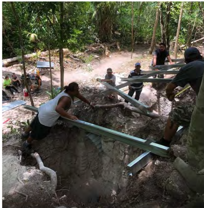
Figure 2.8. Construction of zinc roof over excavation area (Haines 2019).
